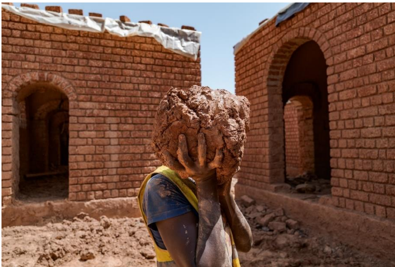
At the Morija clinic in Kaya, a place to the north of Ouagadougou, workers craft a curved “Nubian vault” structure, designed to keep interiors cool. The earthen building will be Burkina Faso’s largest of its kind.
