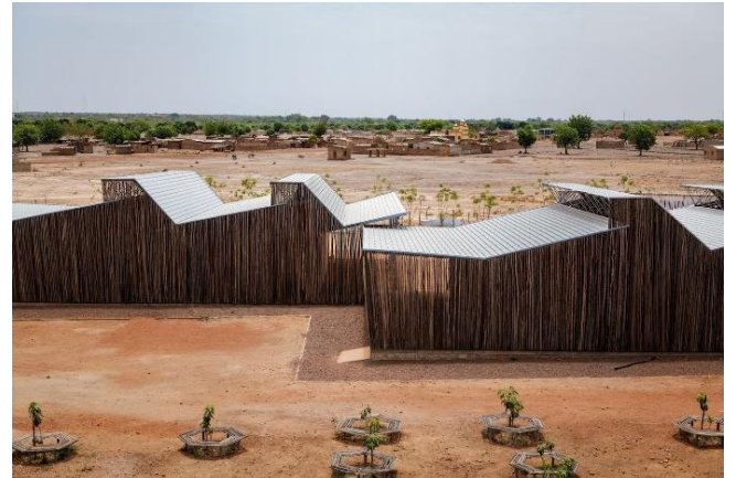
At the Burkina Institute of Technology in Koudougou, designed by celebrated Burkinabe architect Francis Kéré and completed in 2020, poured clay forms the massive walls. A facade of eucalyptus wood creates shade. Above each classroom, a vent allows hot air to escape.
